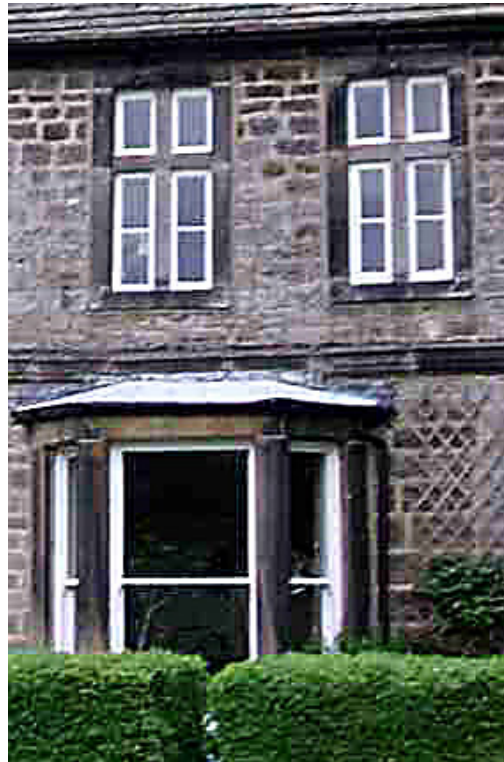
Weston Grange: one elevation, two different eras, two different window types. At first floor the mullioned and transomed casement windows are original to this late seventeenth century building. The large single paned sash windows were inserted in 1890.
