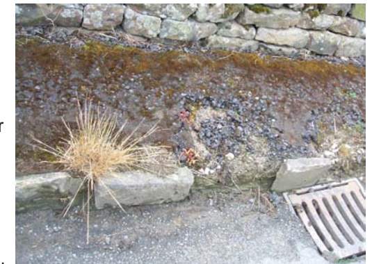
Kerb repairs needed.
