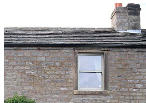
Vertical sliding sash window.
