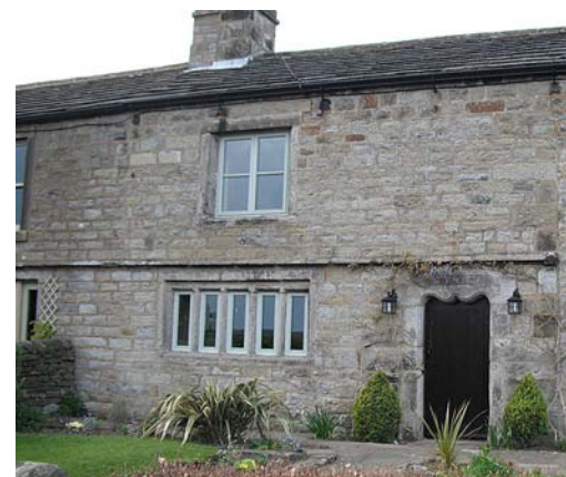
Casement window above mullioned window.
