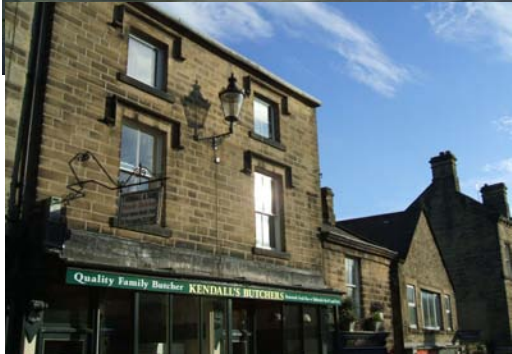
Prominent Buildings on High Street.
