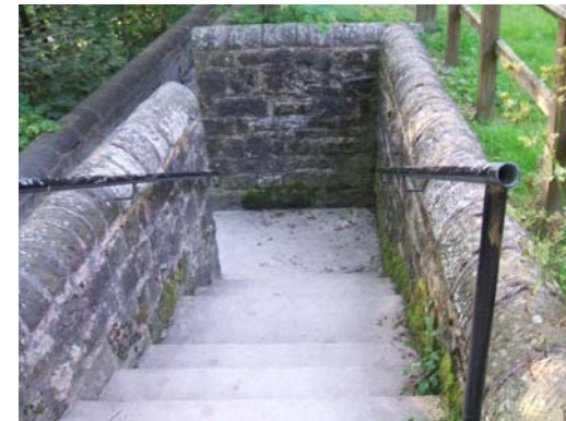
Coursed stone walls.
