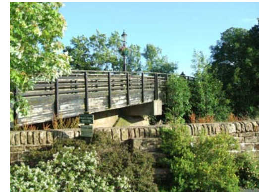
Pedestrian Bridge as seen from from Mill Lane.
