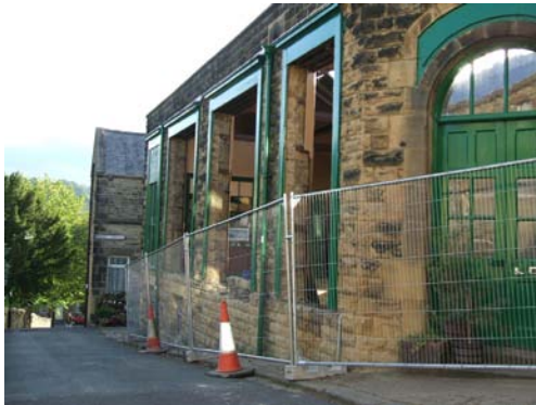
The former Market Hall recently a Car Showroom before demolition.
