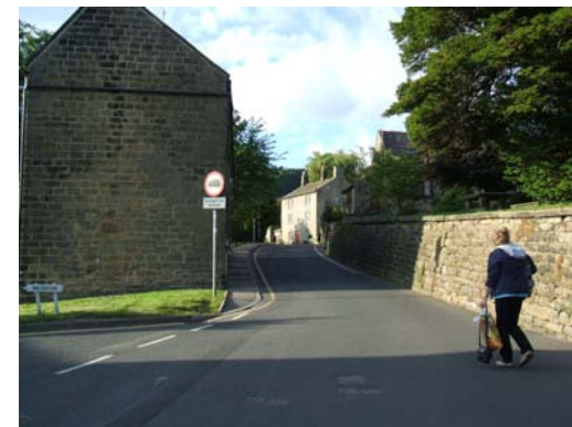
Retaining wall to St Cuthberts Churchyard.
