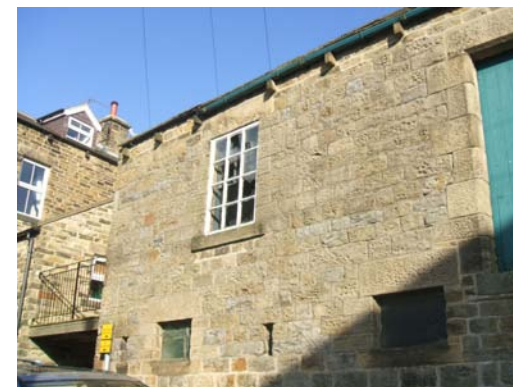
Typical stone detailing.
