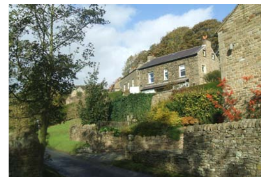
The use of gritstone and sandstone for buildings and boundary walls unites the differing buildings and structures in Nesfield.
