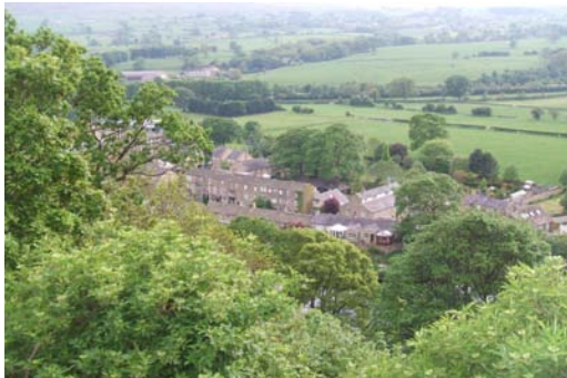
A bird's eye view of Addingham Low Mill village from Castleberg.
