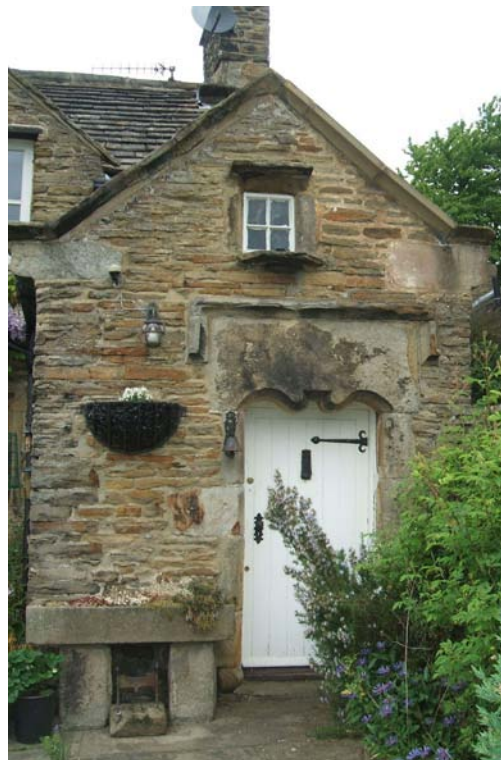
The shallow, irregular coursed local gritstone gives the older buildings in Nesfield a distinctive appearance.
