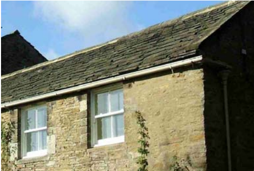
Plain eaves and tabled gables are typical features of buildings in Nesfield.
