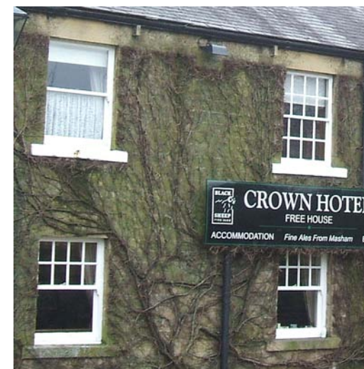
Sash windows through the ages: a Georgian-type sash (top right), a later Victorian sash (top left) and stylish Edwardian sashes (lower windows).
