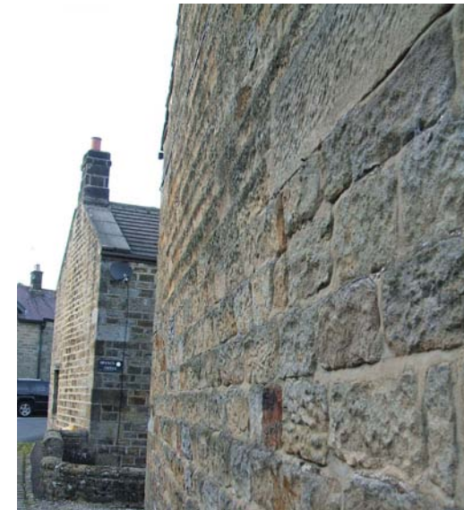
Watershot masonry is a Pennine detail.
