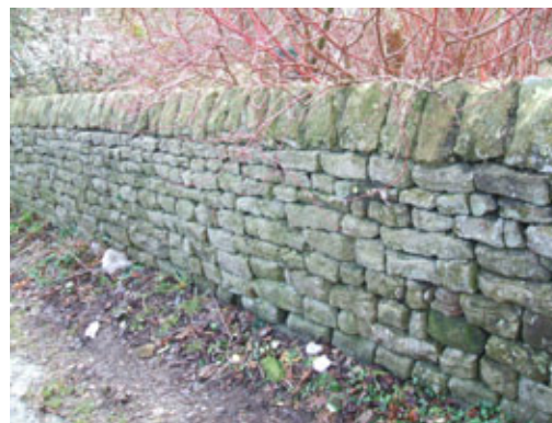
Capped dry stone wall.
