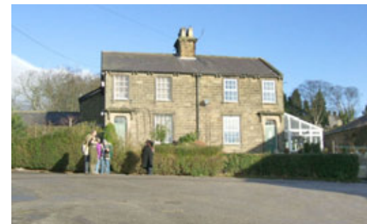
Holm Lea and Mill House adjacent to Glasshouses Mill with Vertical timber sliding sashes (left) and PVCu (right) showing how different fenestration materials affect architectural character.
