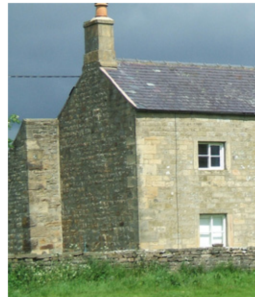
The formal front elevation has smoothed stone, the less important side elevation is faced with less dressed stonework
