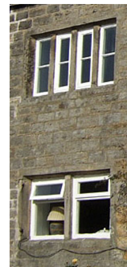
An example of an eighteenth century mullioned window (top) and the same opening, but with two of the mullions removed (bottom) to create large openings which are suitable for sash windows.
